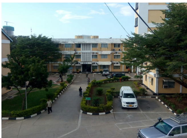
Figure 1: OUT Headquarters in Dar es Salaam
